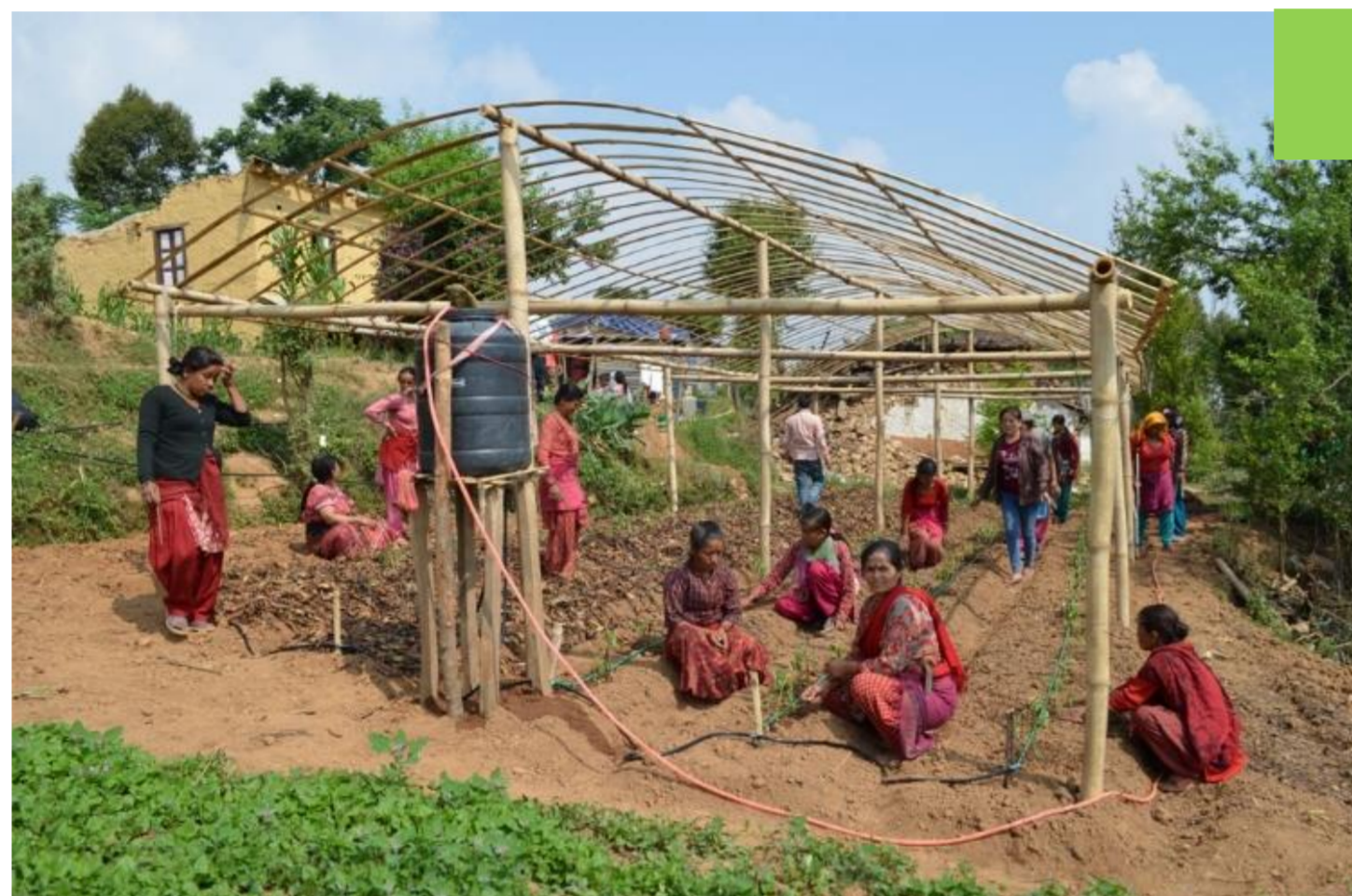
Provision of drip and tank
