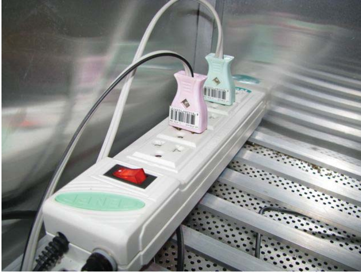
Figure 5: Power strip assembly receiving lead-wires from florescent tube assemblies.
