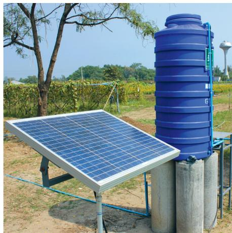
A solar-powered pump — shown here at the Horticulture Innovation Lab's Regional Center at Kasetsart University—can enable drip irrigation in remote locations, where access to electricity, high costs of securing fuel, and distance from a water source can make irrigation prohibitively difficult for smallholder farmers.
